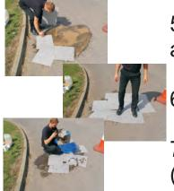
5. LAY 8 absorbent pads on treated area to absorb the oily emulsion.
